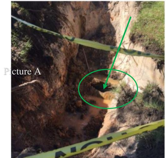
EXISTING 18" CAST IRON SEWER PIPE BREAK
