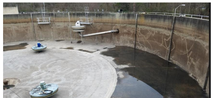
Figure 3. North Tank after cleaning
